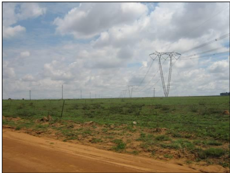
Figure 5: Land use along the western corridor within the ELM
